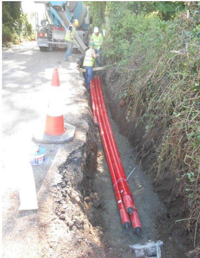
Plate 3-8: Cable Duct Laying in Trefoil Configuration
